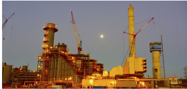
Figure 3: Combined cycle power plant utilising high purity water for high purity steam product for a process
